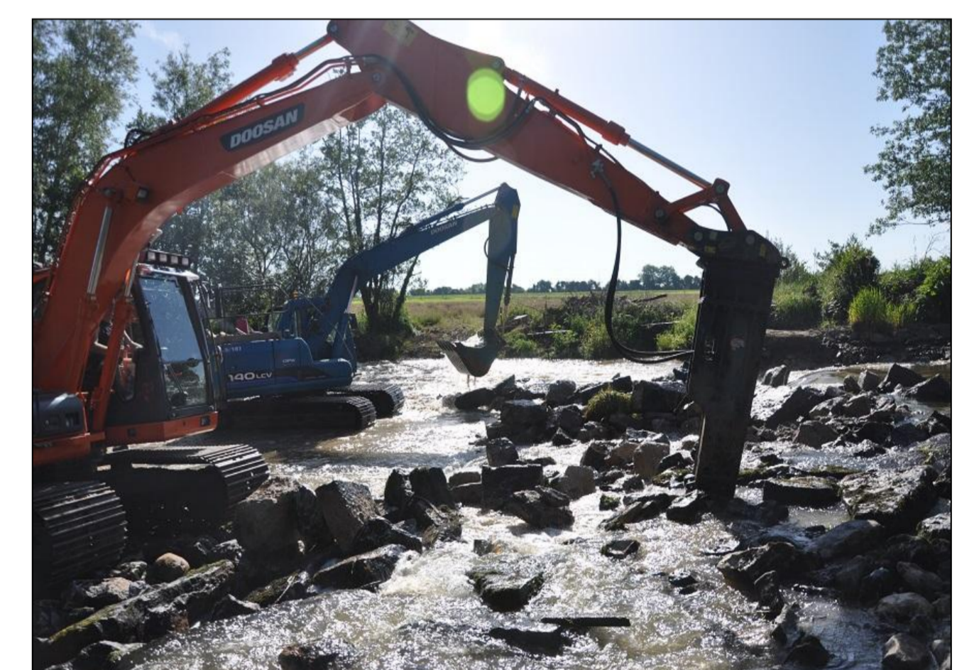
Weir Removal, Ballyclogh, Mulkear River, Aug. 2013
